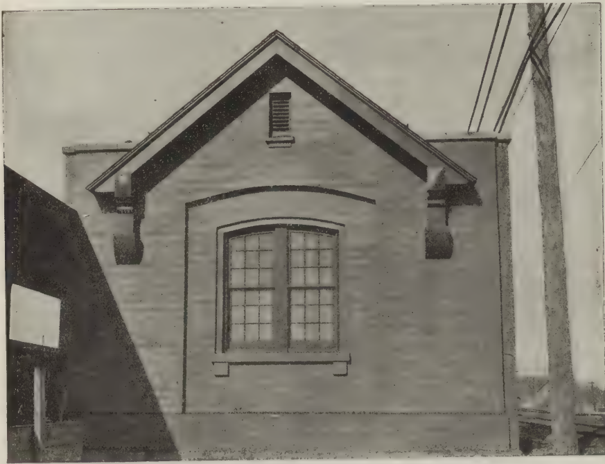
FIG. 31.—Rubbed concrete surface treated with cement stain. Special mortar facing.
